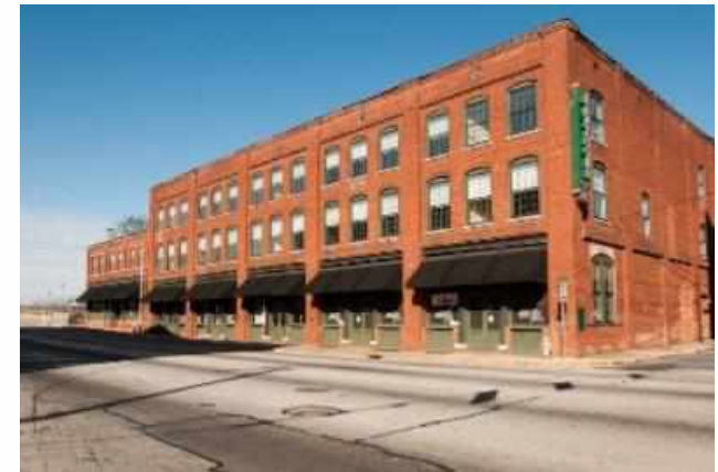
Historic building in Downtown Rome, Ga readapted as a hotel
